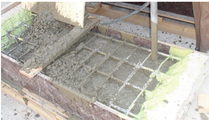
(b) Placing of the repair concrete
