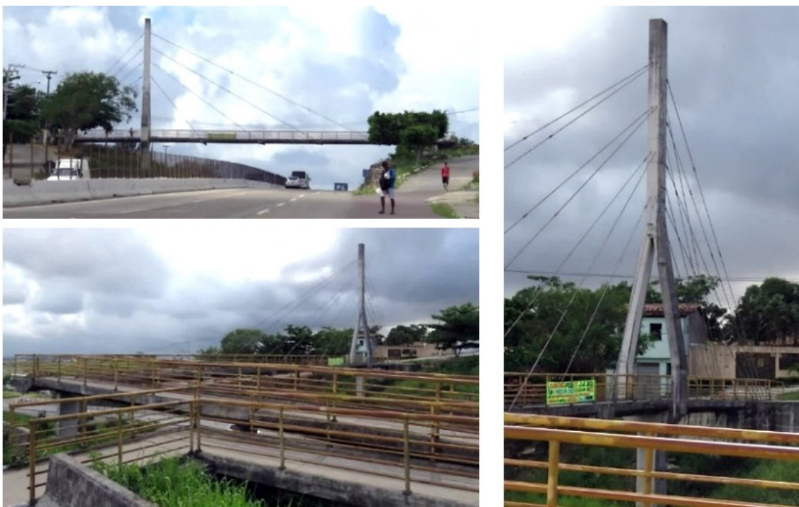
Figure 1 Cable-stayed footbridge in Sergipe, Brazil.
