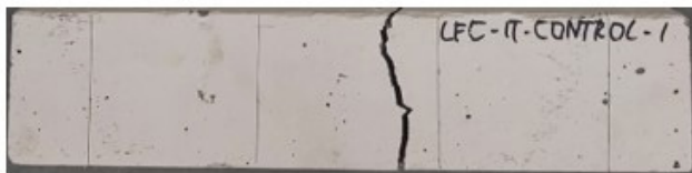
(a) Flexural failure Control concrete
