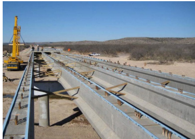
Figure 3. Temporary wooden cross-frames in Live Oak Bridge in Texas. Source:(PCI, 2011).
