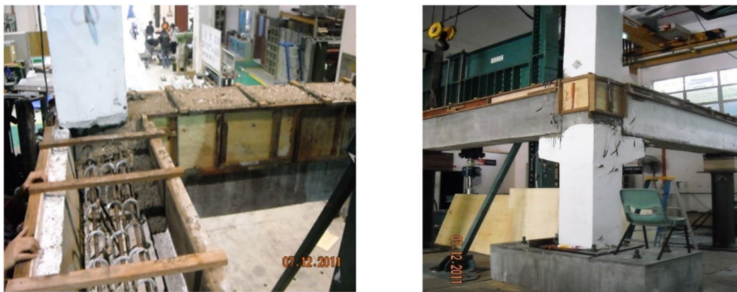
(a) construction of in-plane and out-of-plane beam and top column (b) corner beam-column joint placed on top of the foundation beam
