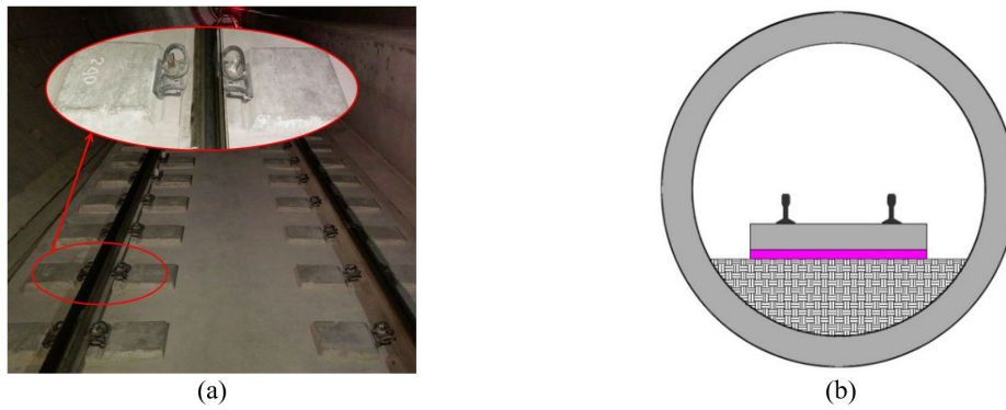
Figure 4 Views of the superstructure of slab track in the field test: (a) View of slab track; (b) schematic view Floating Slab Track (FST).
