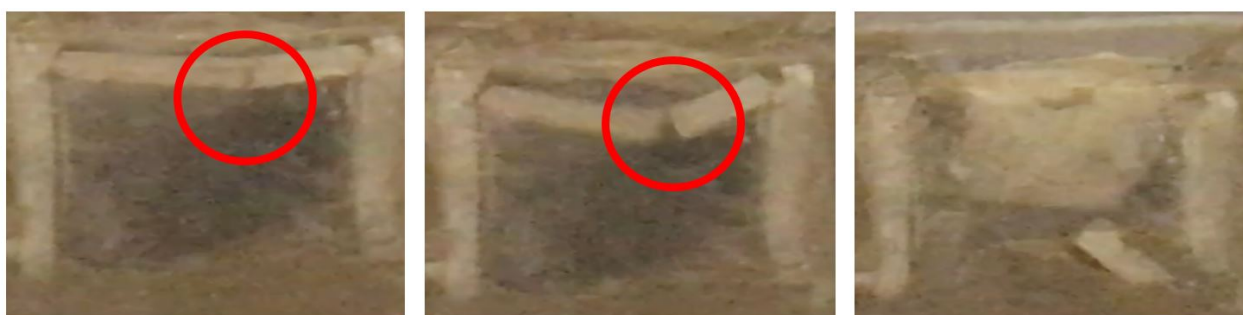
(a) Plastic failure of the utility tunnel before foundation reinforcement
