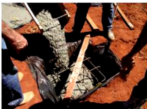
Figure 9 Pouring the concrete for DPR_{(EXP)} .
