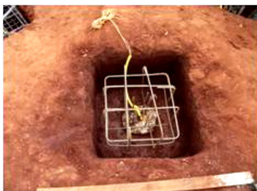
Figure 8 Positioning the reinforcement for DPR_{(EXP)} .
