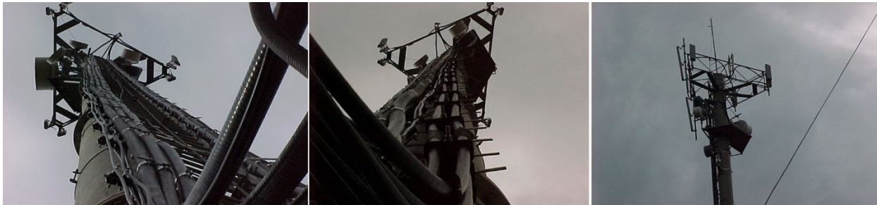
Figure 3. Pictures of the reinforced concrete pole
