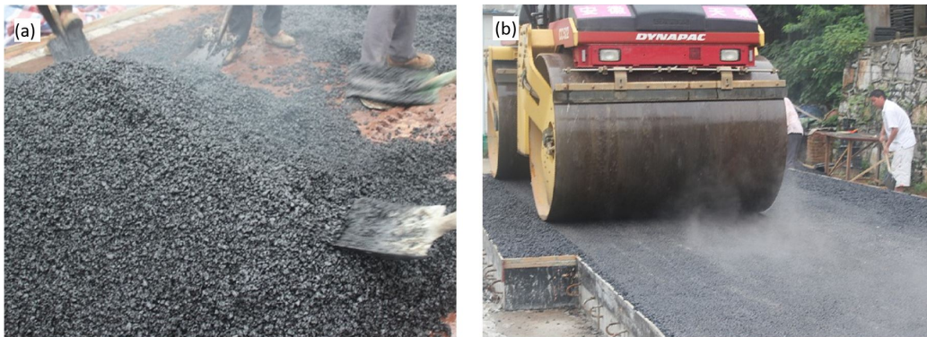
Figure 3 Test site: (a) the paving process of SMA; and (b) the rolling process of SMA.
