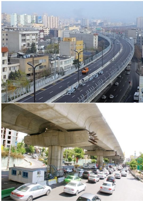
(a) Photographs of Sadr Bridge
