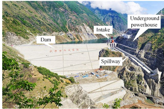
Figure 4: Downstream view of the Pubugou hydropower station.
