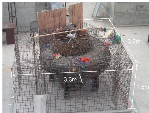
Figure 6: Reinforcement layout of the PFSCS.
