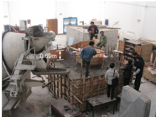
Figure 7: Field-pouring of the SMC.
